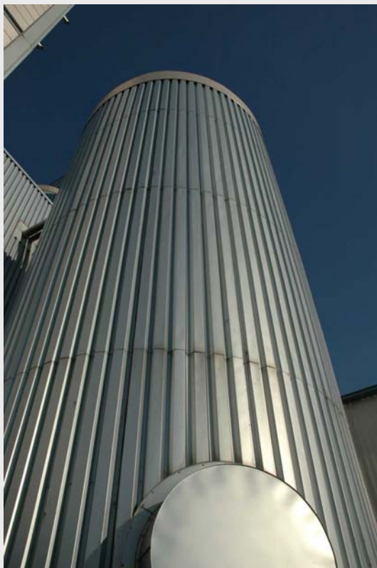
CO 2 Storage Tank 90 to
